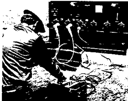
Figure 26. Testing a Cable.
